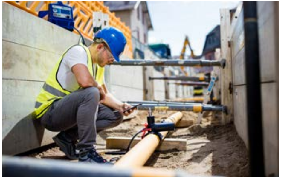
Electrofusion fittings and fusion units for pipe jointing
