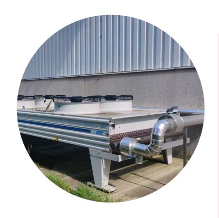
Installation of the free-cooler
