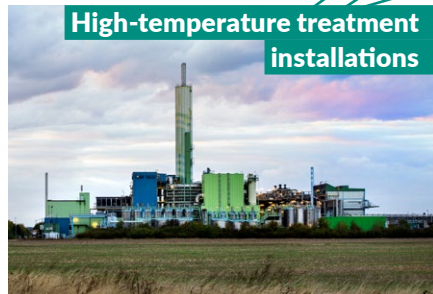
High-temperature treatment installations Specialised high-temperature treatment installations offering safe solutions for hazardous waste. Hamburg (DE) - Biebesheim (DE) - Antwerp (BE)
