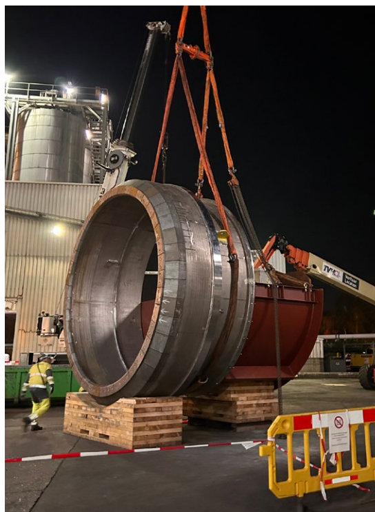
A rotary drum in one of our kilns is being replaced.
