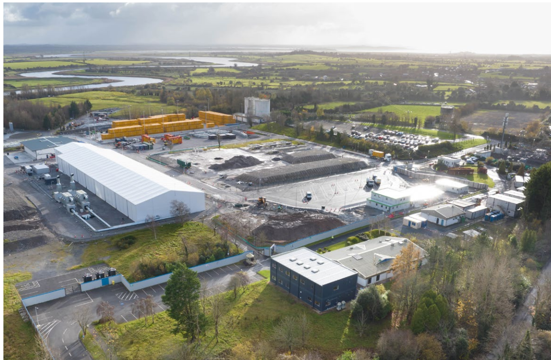
Advanced shelter is crucial for remediation of pharmaceutical site.
