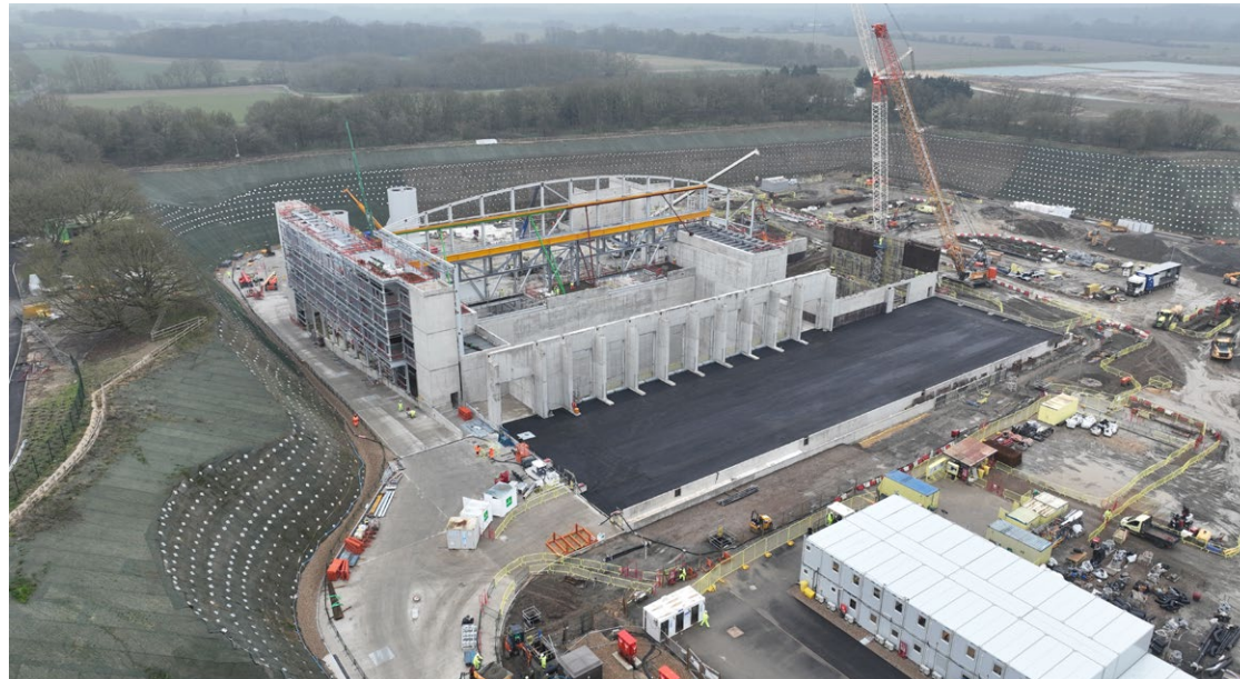
Our largest treatment installation to date is rapidly gaining shape.
