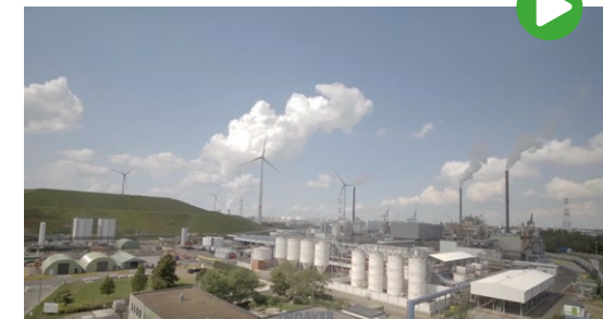
Behind the screens of the construction of Antwerp North Heat Network
