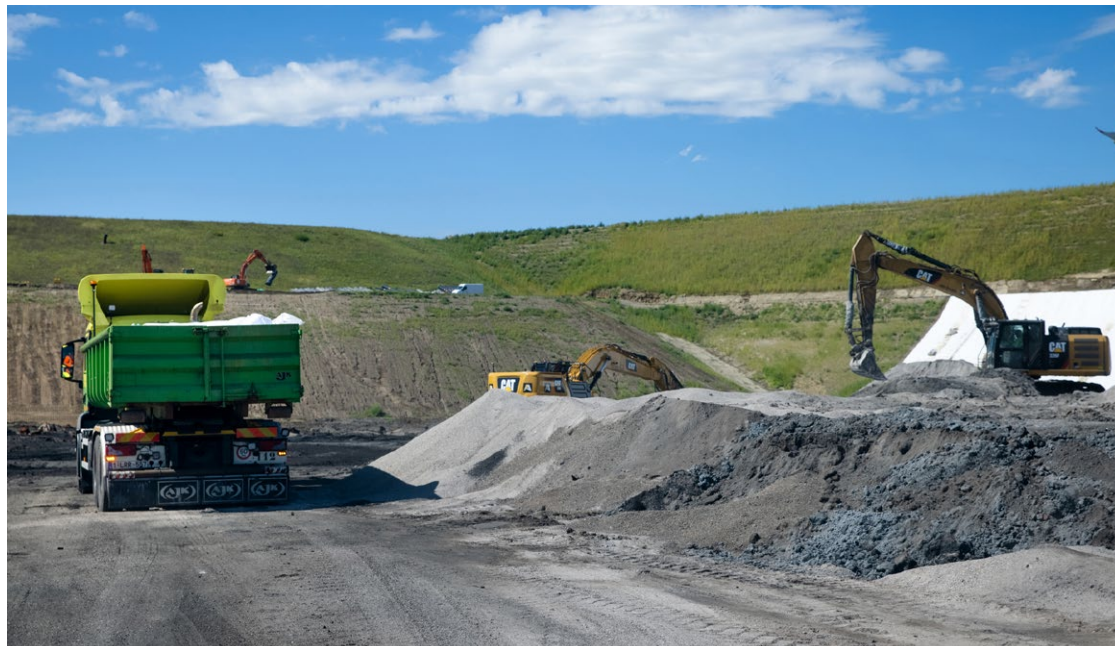
Hazardous waste at one of our landfill sites.
