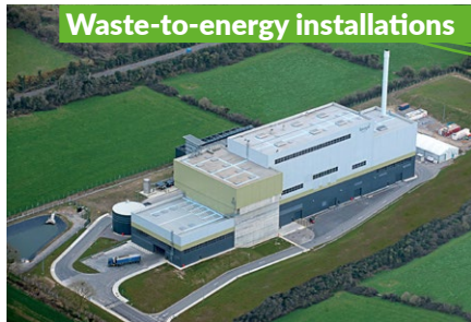
Waste-to-energy installations Large-scale waste-to-energy installations for valorizing energy from non-recyclable waste streams. Doel (BE) - Meath (IE) - Aberdeen (UK) - Rivenhall (in construction, UK)
