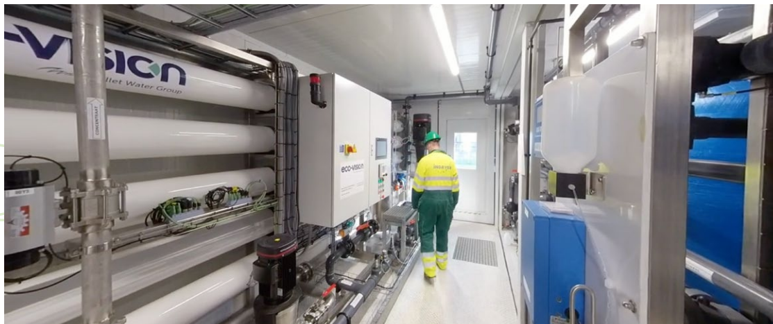
Reversed osmosis to further clean the waste water.
