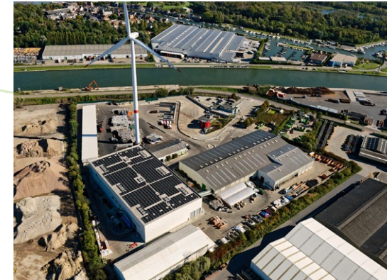
Willebroek (BE) counts on the sun and the wind for its energy supply.
