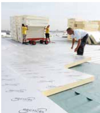
Roof insulation (flat and pitched roofs)
