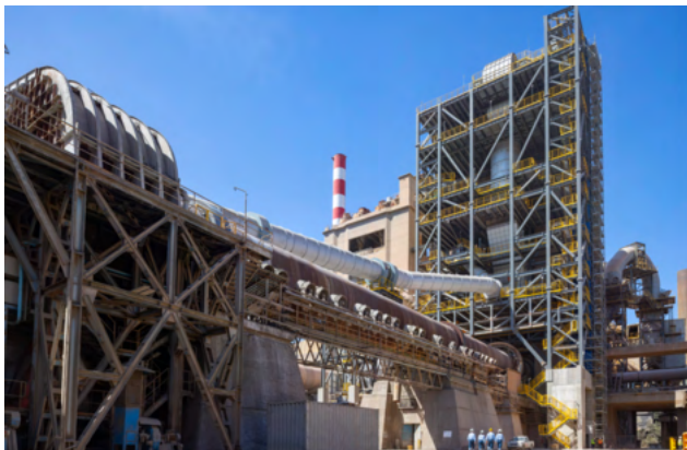
Precalciner unit at Kamari cement plant, Greece.
